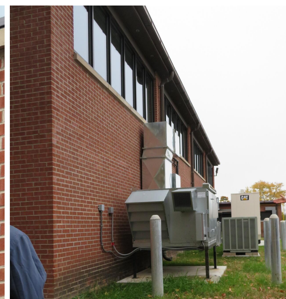
Figure 9: Windows & New Wall Penetrations in West Wall
