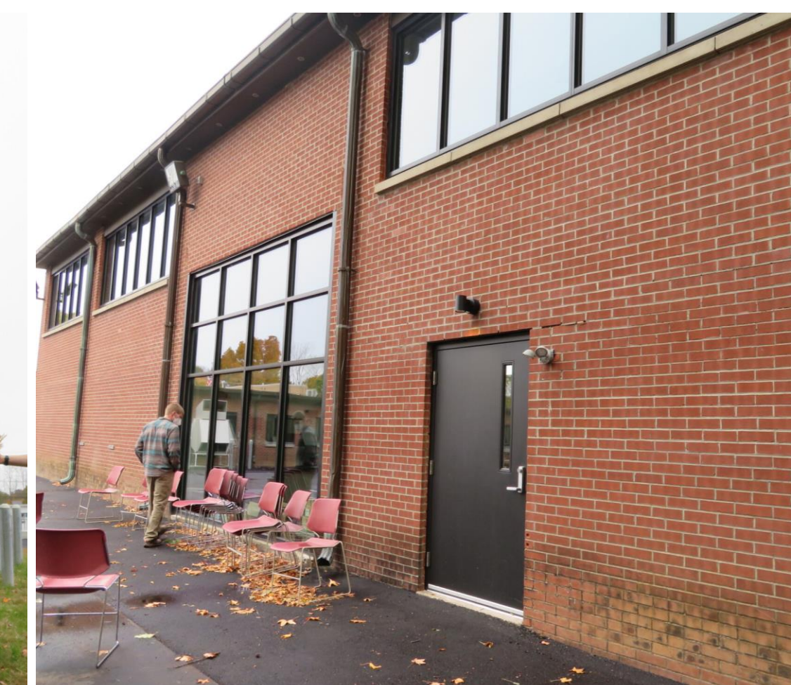
Figure 10: Windows Along East Wall
