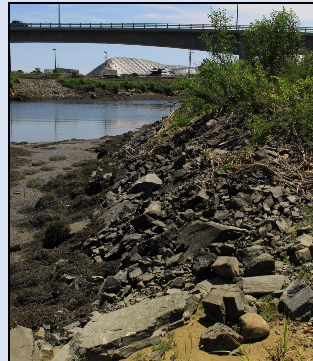
Shoreline armoring with riprap in Cutts Cove from 1980's. Armoring converted fringe salt marsh to mudflat.
