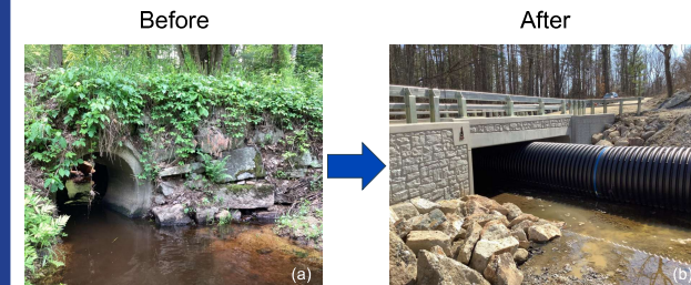
Fig. 4: Culvert in Barrington where we conducted field measurements. (a) Prior to reconstruction, this culvert regularly backed up and overtopped during large rain events. 2023 archive photo by NHGS. (b) Following reconstruction, the culvert tripled in size and was reinforced with wingwalls. The black pipe was a temporary redirection of flow and will be removed following construction. Photo by Connor Paul.
