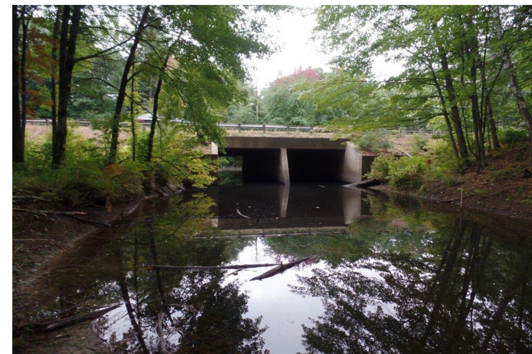
Image #3 Existing Condition of Bridge
