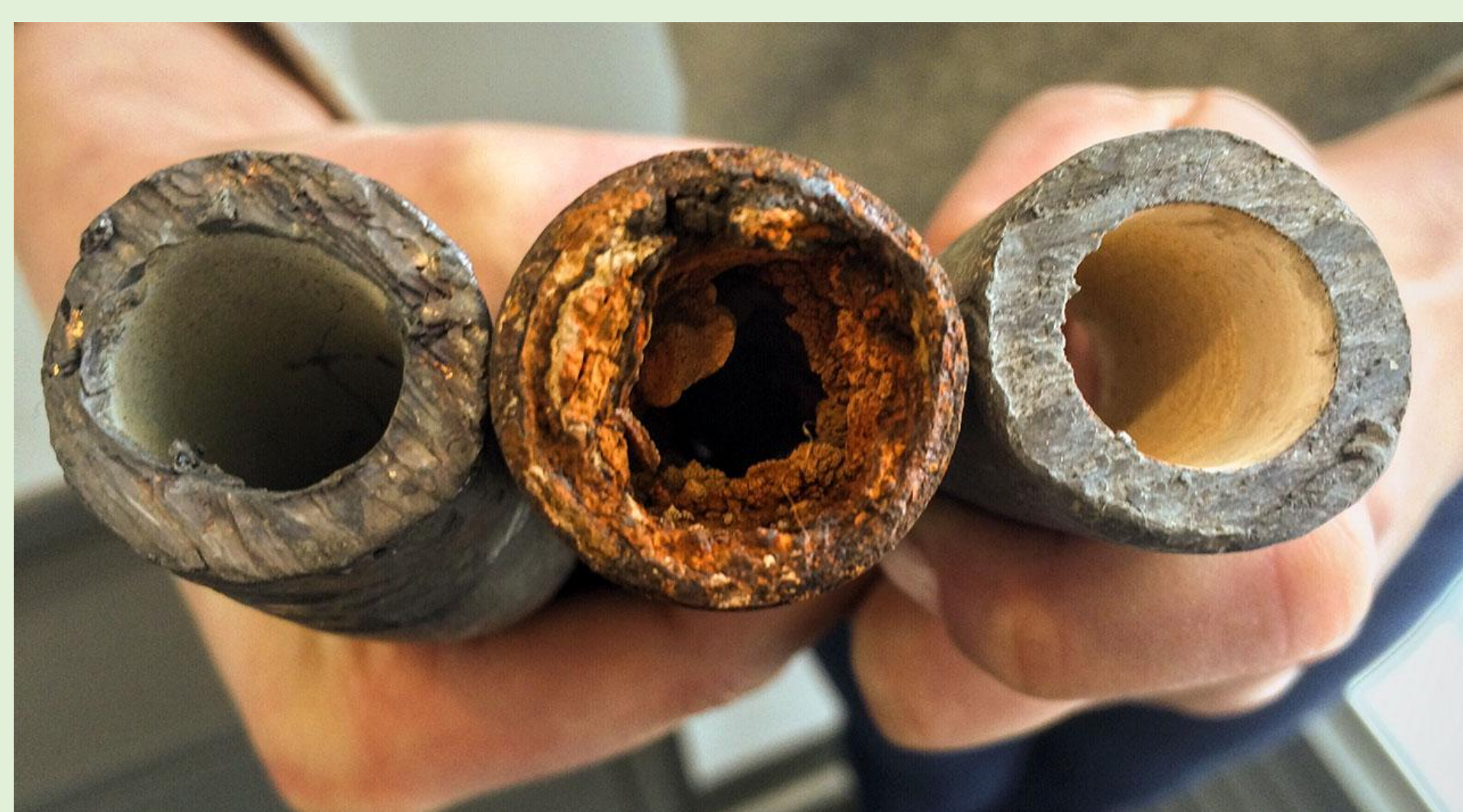
Comparison of new (left), untreated (middle), and orthophosphate treated (right) lead pipes.
