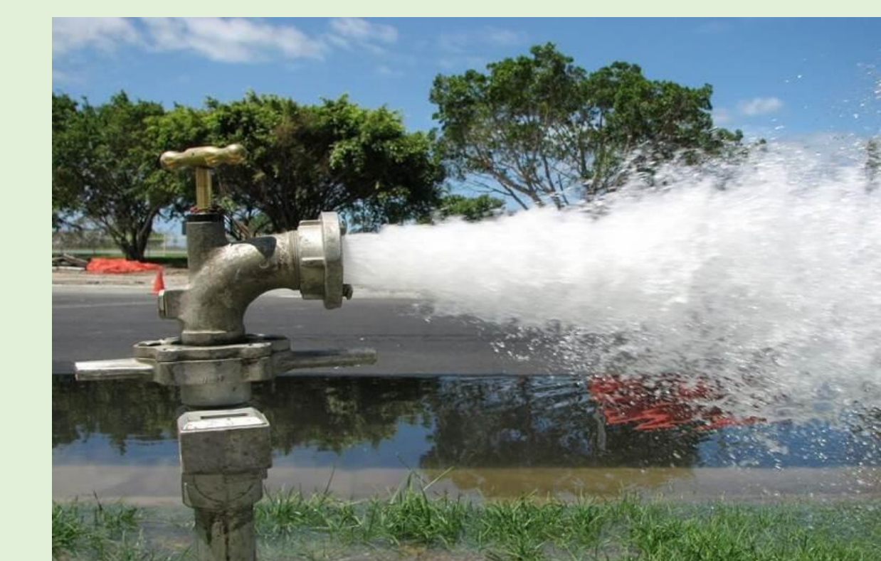
Pipe flushing
