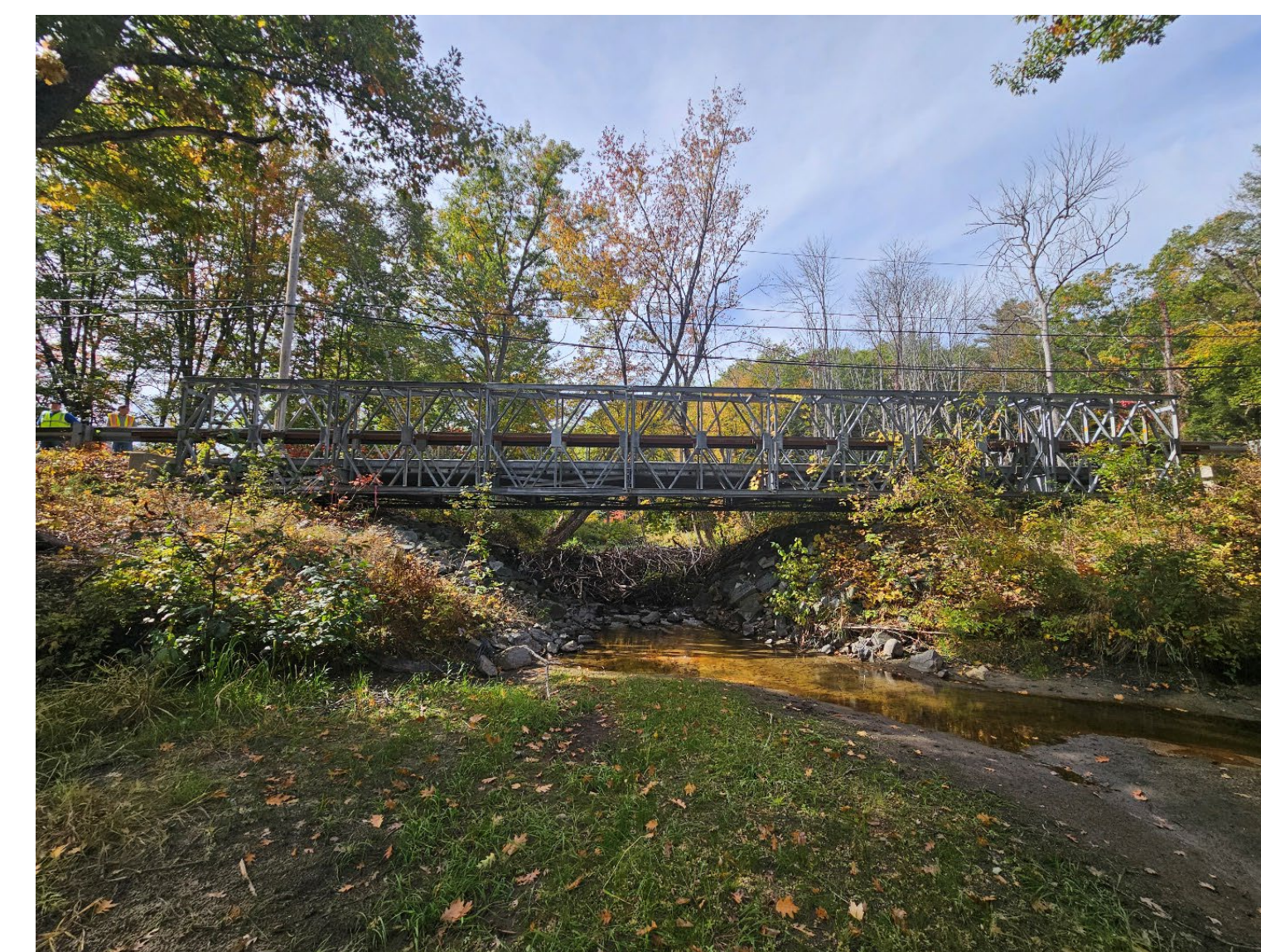
Image #1 Current State of bridge over Knox River
