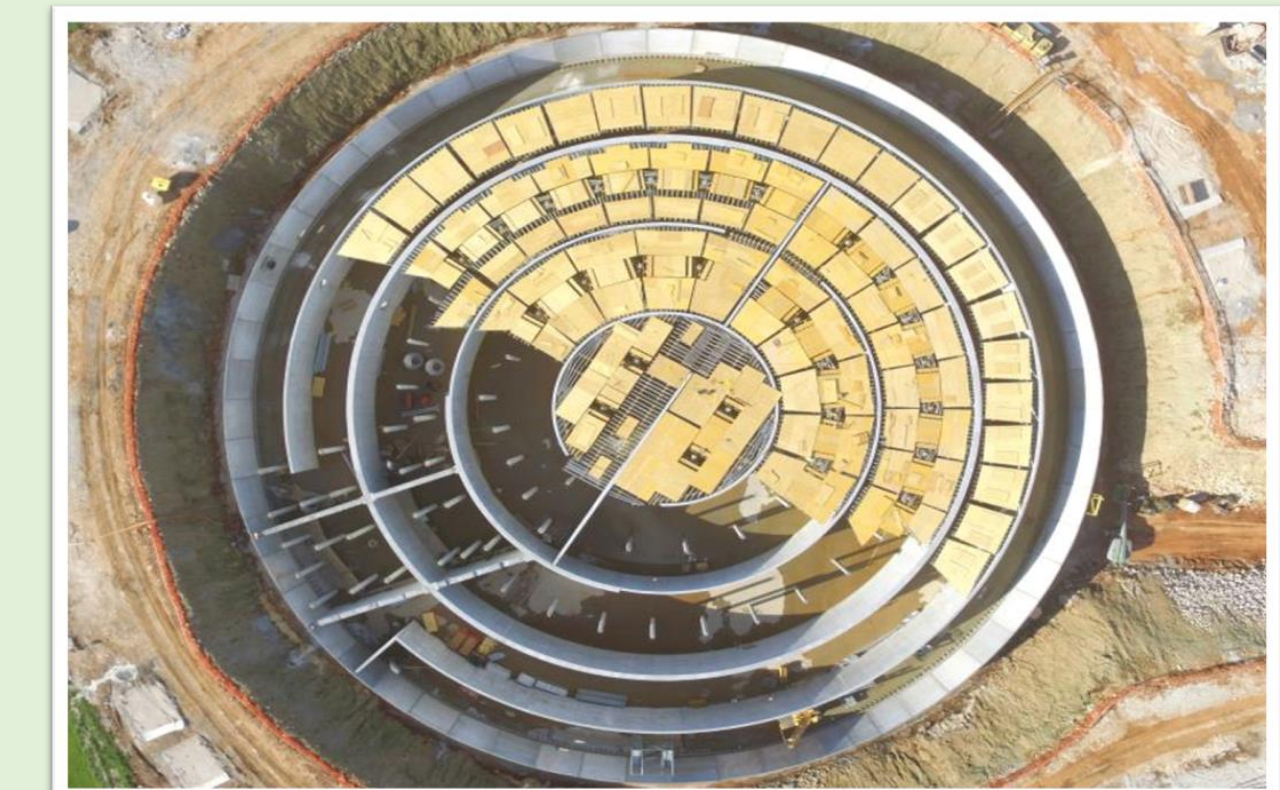
Figure: Tank-within-tank Clearwell Design
