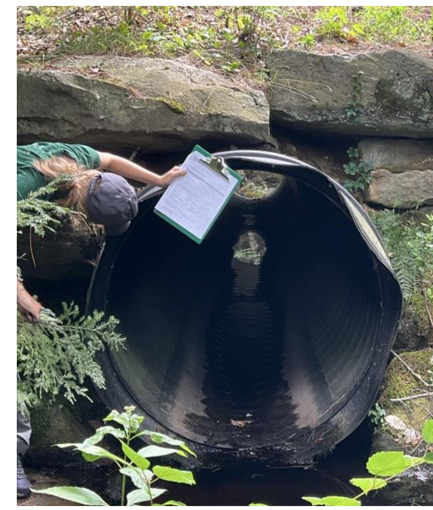
Fig. 2: Lauren checking a culvert for line of sight (LOS).
