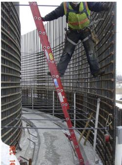
Figure 15: Existing radial reinforcement.
